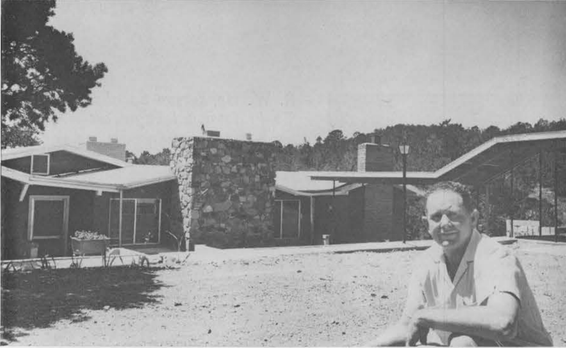
SPRAWLED ON A HILLSIDE in the Sandia Mountains is the 2,400-sq.-ft. house built by Garvis Chandler (4224). The house took six years of spare time work to construct.
